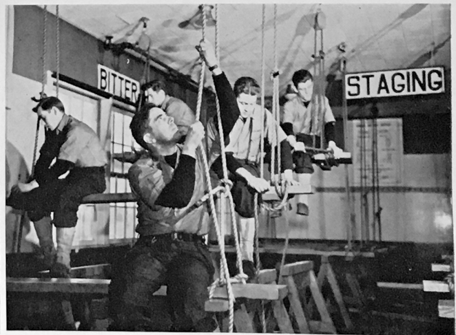
Stagings are rigged by two-man teams.
